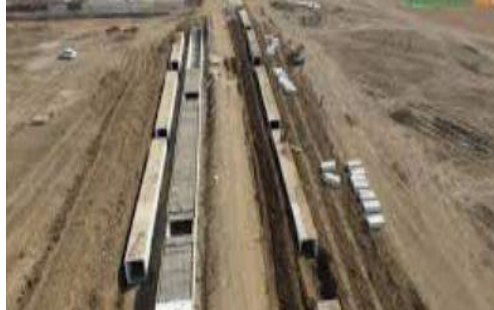
Drainage network construction
